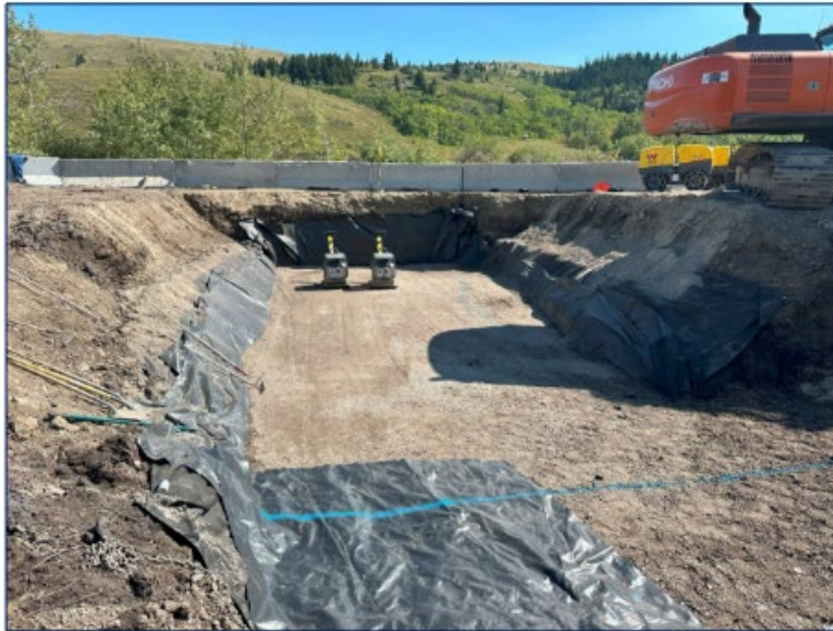
September 8, 2024 Structural base installation is underway.
