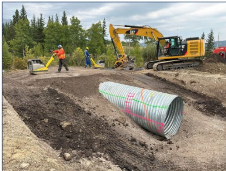
September 11, 2024 Backfill of upstream barrel section completed.
